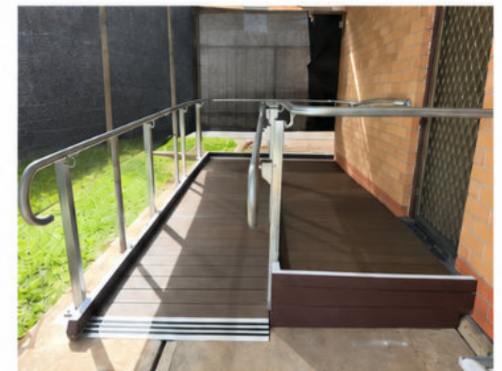
03 Ramp, platform and steps
